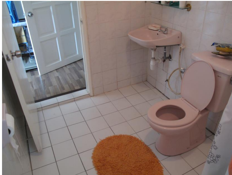
Figure 6. Floor-level lowering of the bathroom (photo by Seo)
