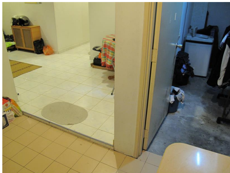
Figure 5. Floor-level lowering from living room to kitchen and to drying yard (photo by Seo)
